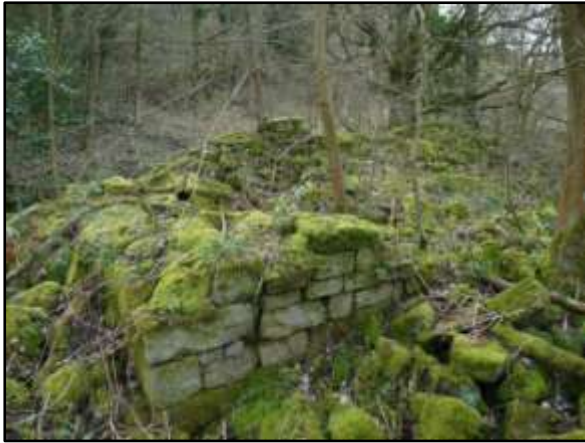
17 North East wall and rear entrance
