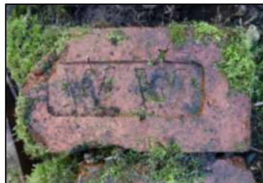
1F Brick from above the cellar
