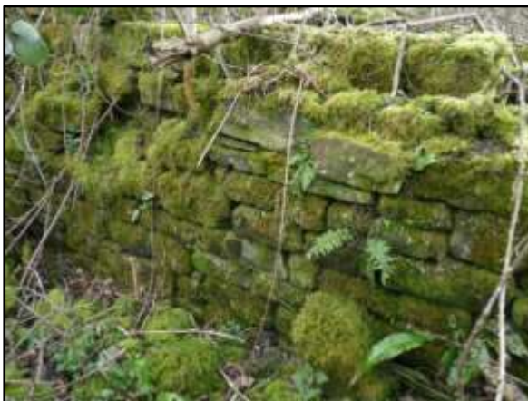
Interior wall 12 Long Barn
