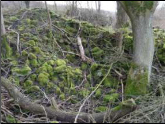
Dividing wall between Warehouses 6A / 6C
