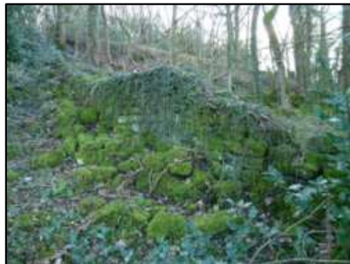
East wall 16 Upper Barn
