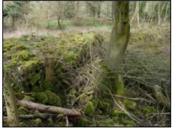
Interior west wall 6B
