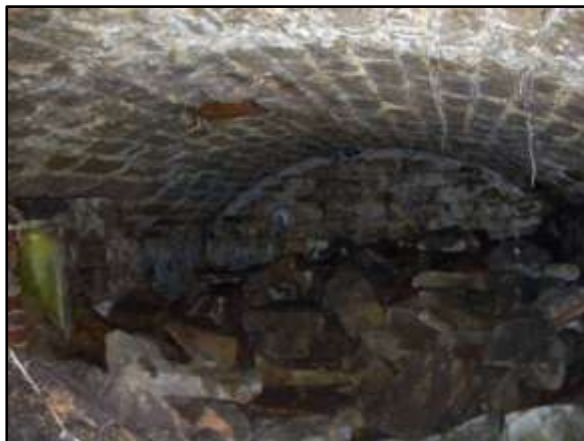
Inside the cellar
