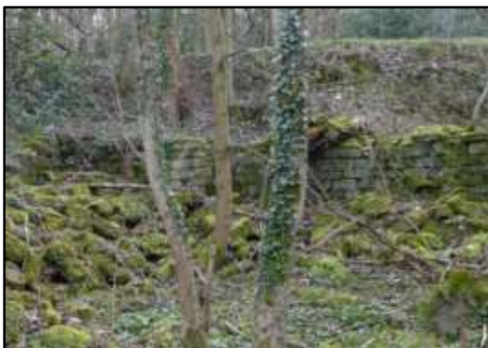
North east wall 16 Upper Barn
