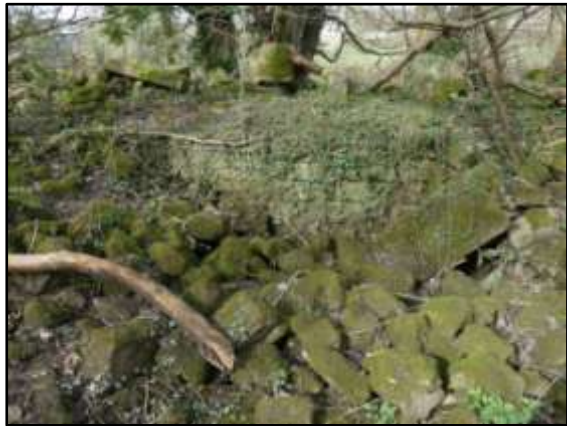
Interior west wall Fulling Mill 8
